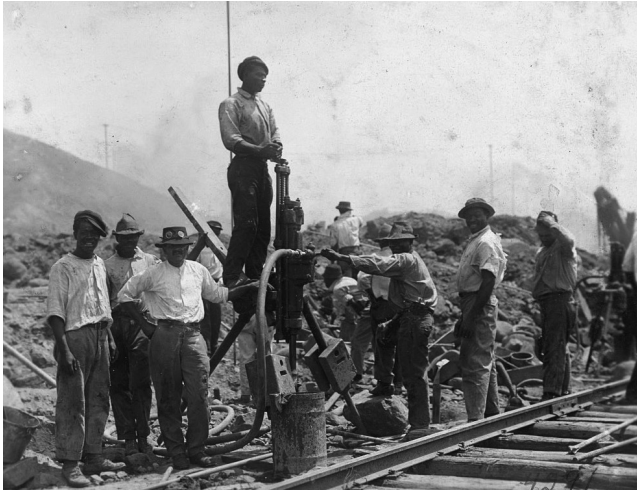
Railway workers with pneumatic drill. Undated photograph.
