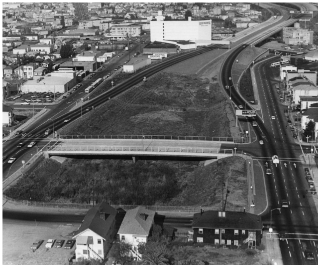
COURTESY OF ROY H. WILLIAMS/MEDIA NEWS GROUP/OAKLAND TRIBUNE VIA GETTY IMAGES Interstate 980 severed the predominantly Black neighborhoods of West Oakland from the rest of the city, setting the stage for underfunding of municipal projects in the area. Excavation site of Interstate 980. (1976)
