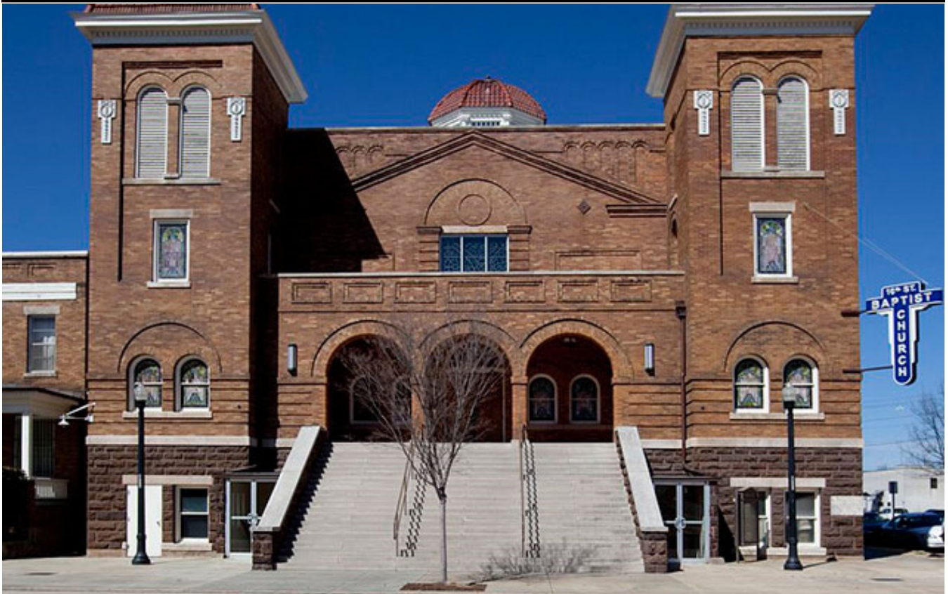
16th Street Baptist Church, Birmingham, Alabama . Carol Highsmith Photo
