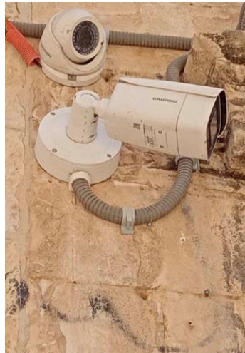
HIKVISION P/T/Z Cam mounted above Grundig bullet cam. © Amnesty International
