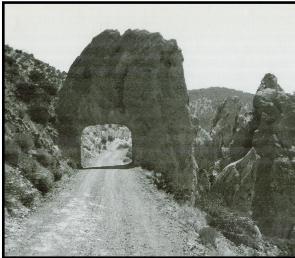
Mule Creek Highway, c. 1922.
