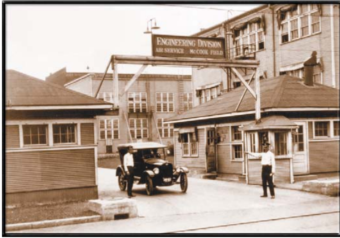
Civilian guards at the main gate of McCook Field.
