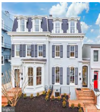
ASI Ministry – Former Home of Frederick Douglass?
