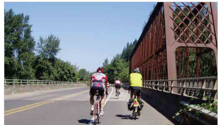
A wide, paved shoulder is an option on a more rural street section.
