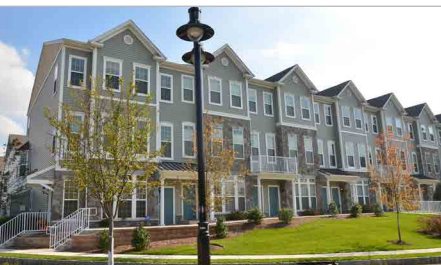
Individual entryways and porches and building articulation can reduce the visual scale of multi-family housing
