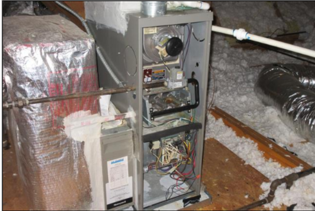
6.0 Item 1(Picture) attic unit
