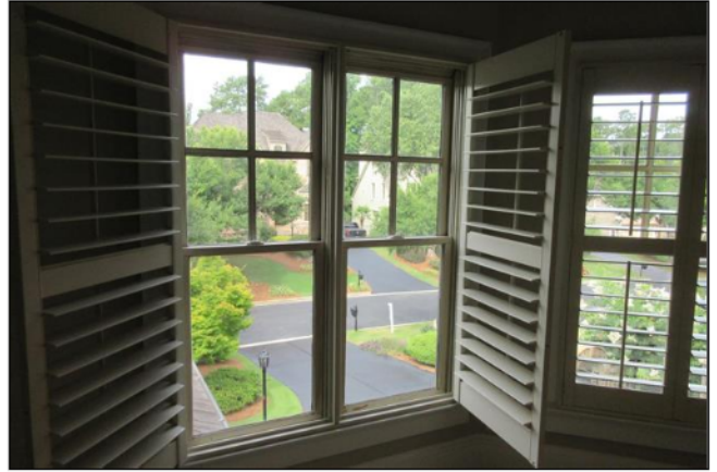
9.6 Item 2(Picture) left front bedroom
