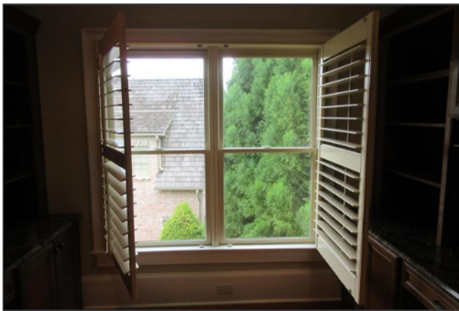
9.6 Item 3(Picture) rear left bedroom
