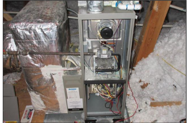
6.0 Item 2(Picture) attic unit
