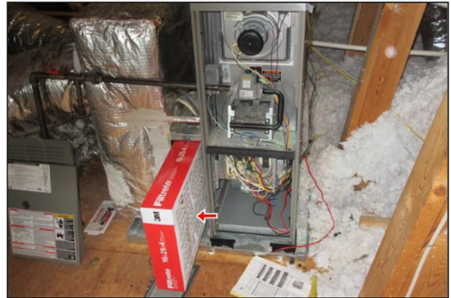
6.2 Item 2(Picture) attic unit
