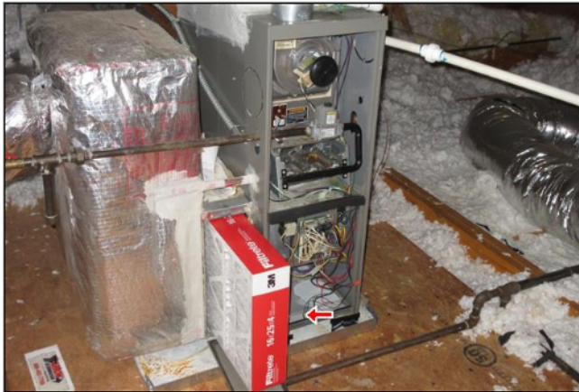
6.2 Item 1(Picture) attic unit
