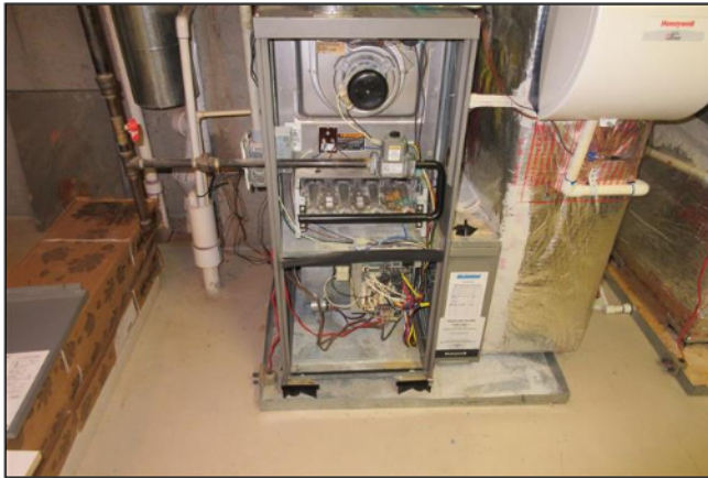
6.0 Item 3(Picture) basement unit
