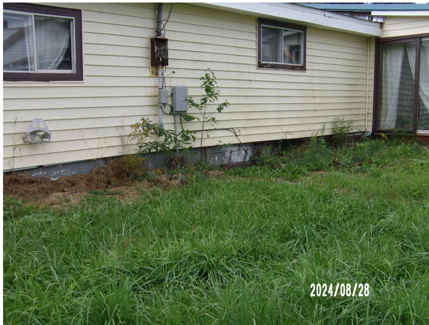
Mortar missing on block foundation on North side of house.
