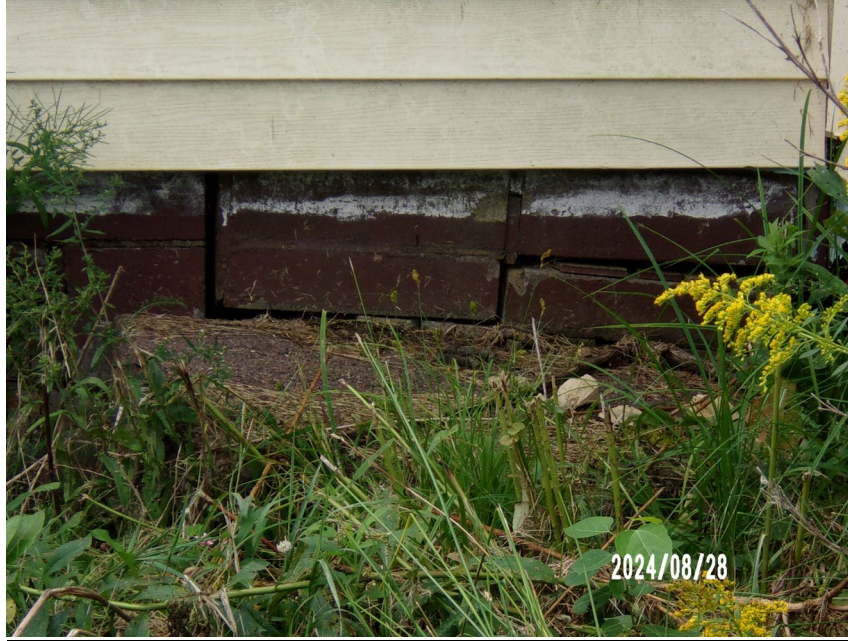
Mortar missing on block foundation on North side of house.
