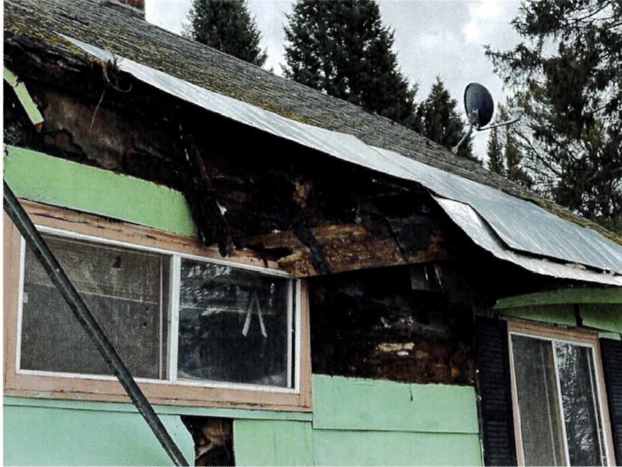
West wall of house.
