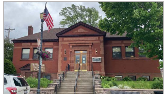
Public Facility - Library
