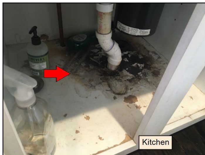
82. Water damage
