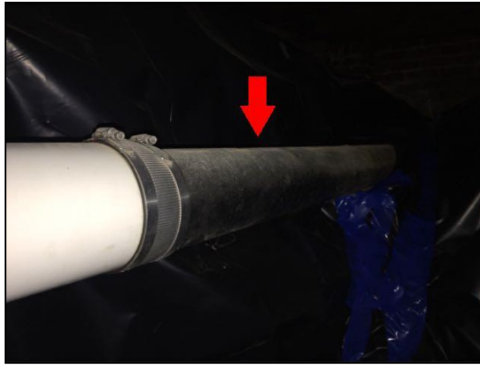
60. Cast Iron drain line is present. This is th...
