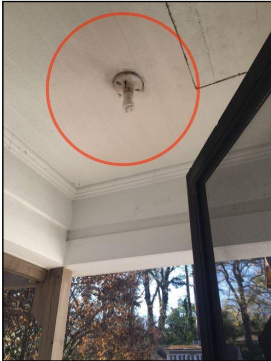
50. Inoperative Task: Repair Time:...
