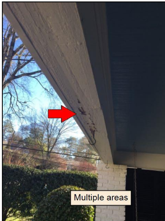
14. Paint or stain needed Task: Provide Time: A...
