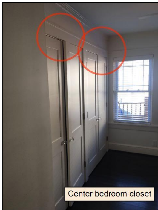
79. Does Not Latch Properly Task: Adjust Time...
