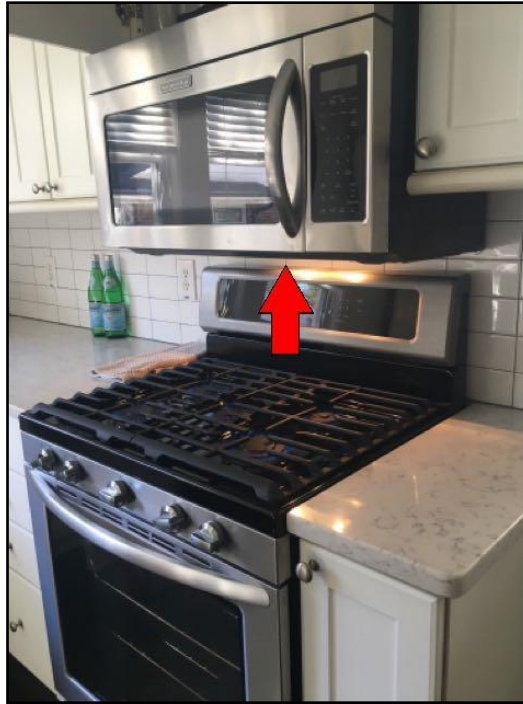
90. Poor clearance
