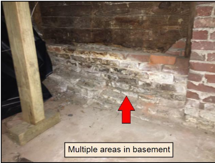
87. Efflorescence
