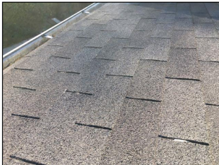
9. Visual inspection from roof surface
