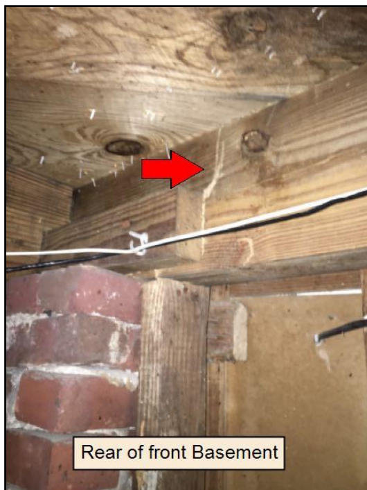
91. There are existing termite "tubes" or...
