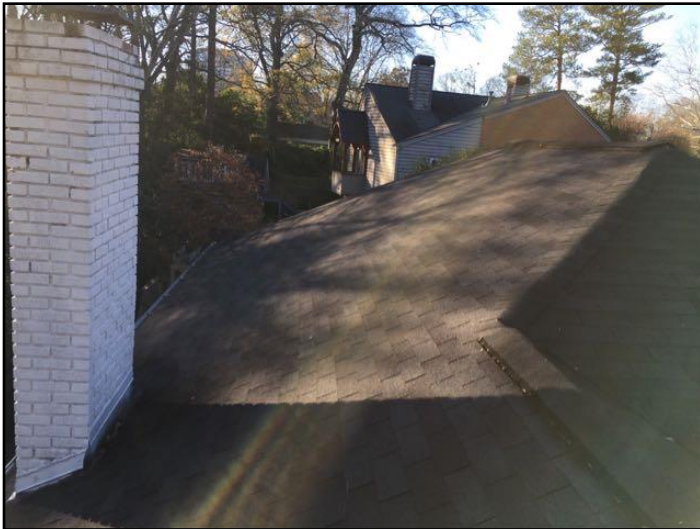
5. Asphalt shingles
