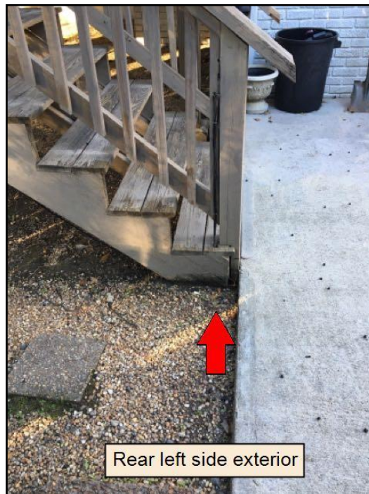
17. Wood/soil contact Task: Correct Time: As...
