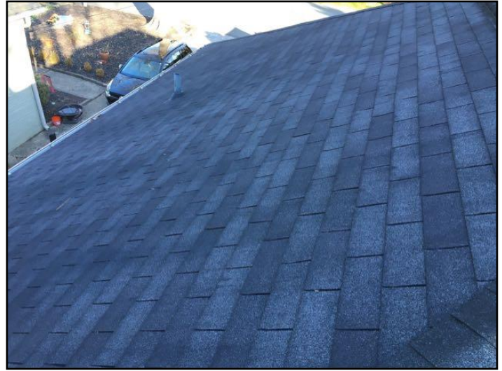
8. Asphalt shingles
