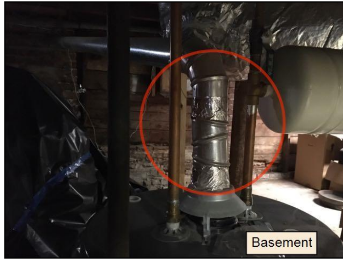
59. Tape not heat rated Task: Remove or replac...
