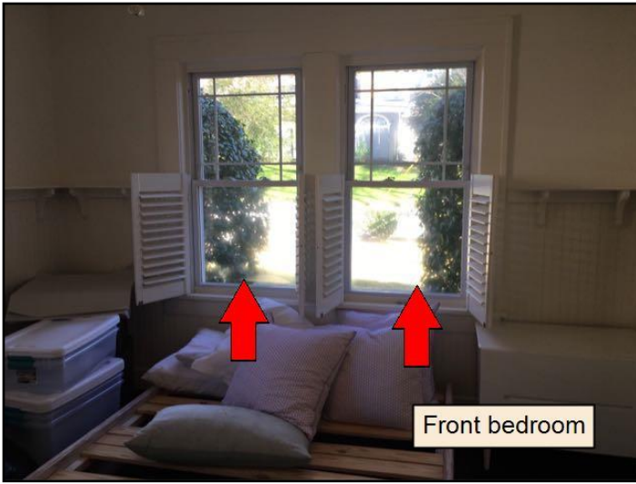
75. Lost Seal in Double or Triple Glazing Task...
