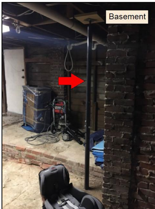
22. Temporary Supports Task: Repair as...
