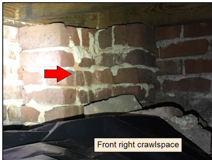
92. There are existing termite "tubes" or...
