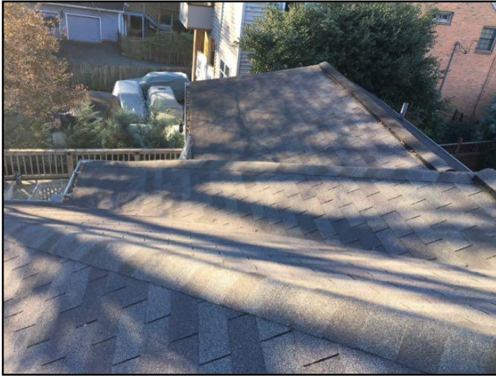
7. Asphalt shingles
