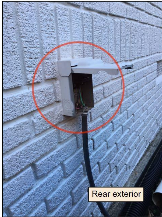
47. Cover loose or missing Task: Correct Time...
