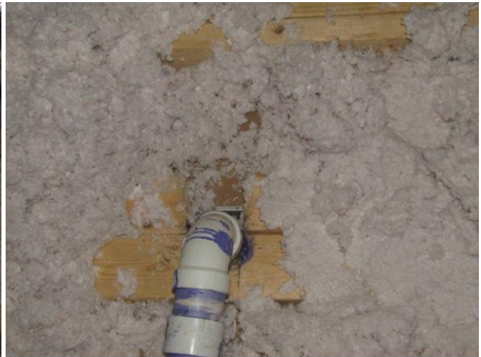
compacted insulation in the upper attic
