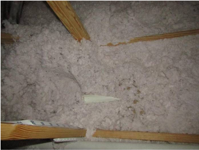
compacted insulation in the upper attic
