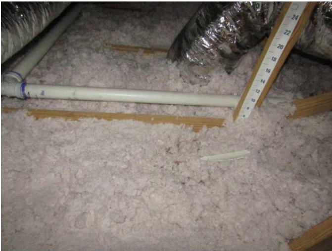
compacted insulation in the upper attic
