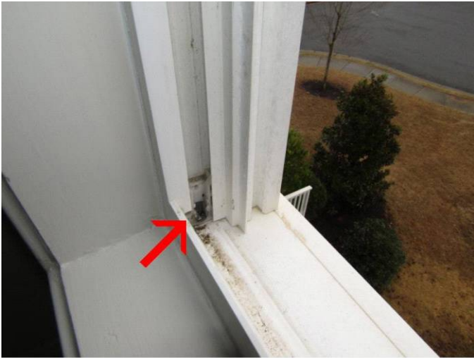
disconnected ballance spring
