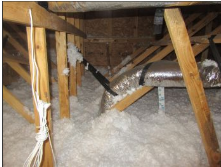
Attic framing and insulation looks good
