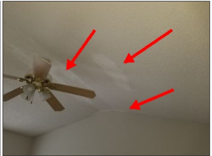
Paint repairs at front guest bedroom ceiling
