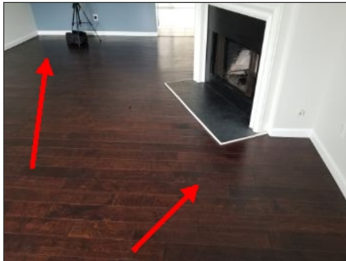
Vertical movement at flooring
