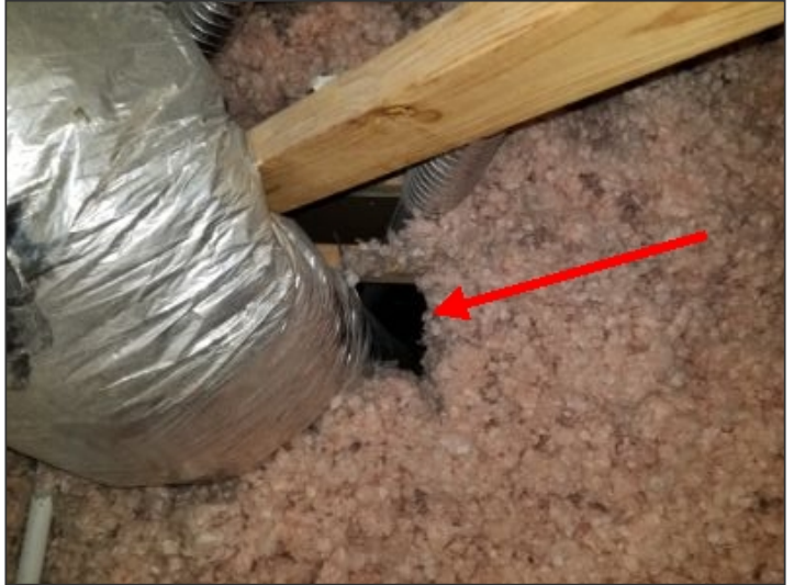
Open chase at attic floor to the right of furnace
