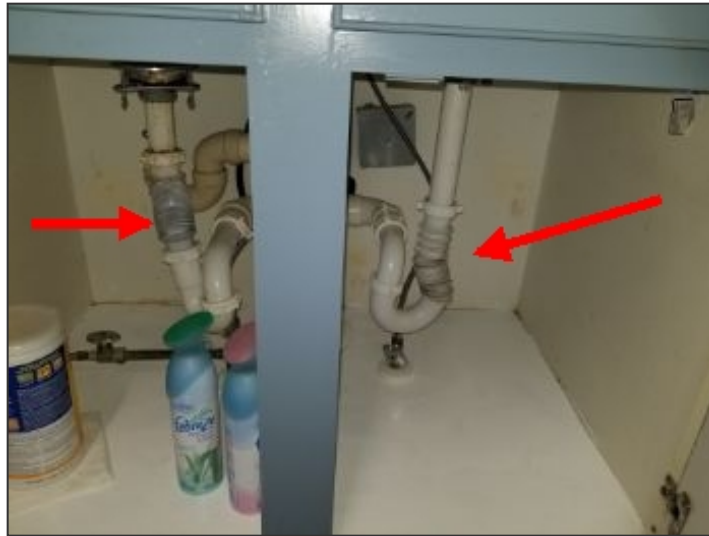
Flex drain lines below kitchen sink
