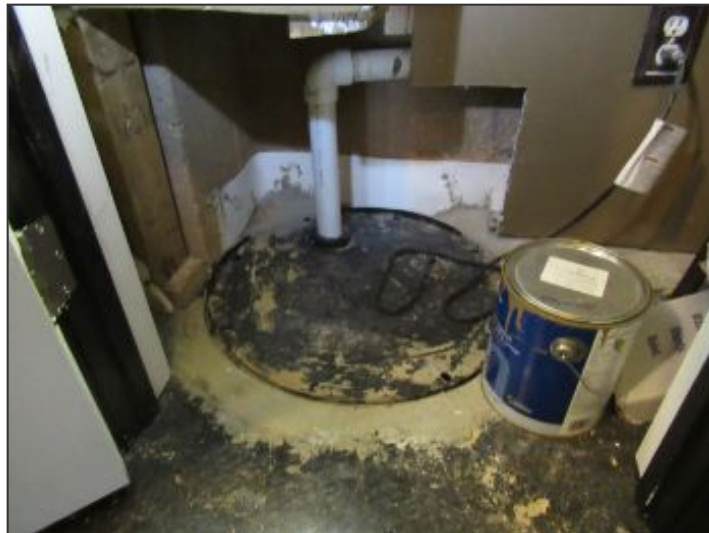
Professional water proofing system at front basement
