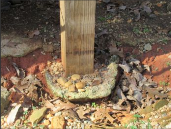
Severe soil erosion at porch support footings Severe soil erosion at porch support footings
