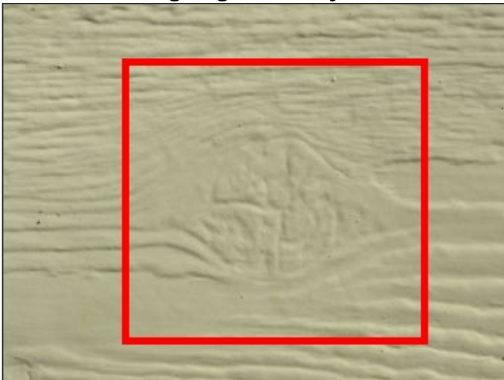
LP signature knot imprint on siding boards
