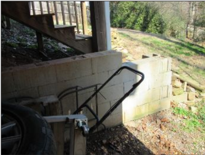
Retaining wall below rear porch
