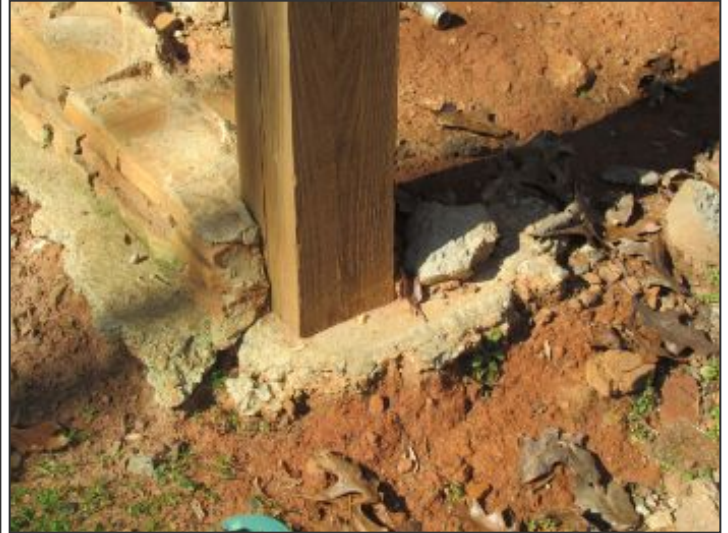
Severe soil erosion at porch support footings Severe soil erosion at porch support footings
