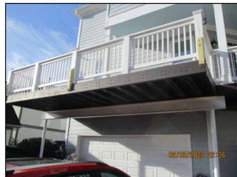
Stairs and handrails are in good condition.
