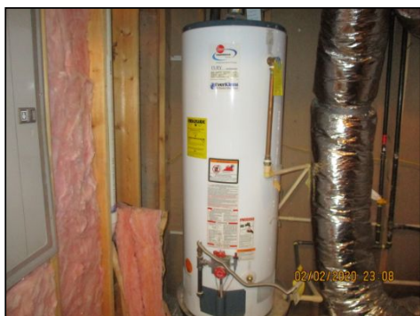
Rheem 2005 gas water heater noted. Unit is nearing the end of its useful life. Recommend licensed contractor to service unit. Be prepared to replace unit in next few years.
