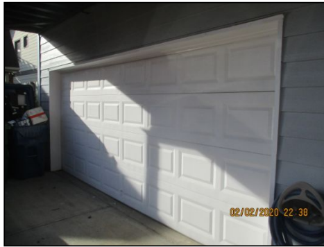
Garage door is in good condition.
