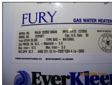
Rheem 2005 gas water heater noted. Unit is nearing the end of its useful life. Recommend licensed contractor to service unit. Be prepared to replace unit in next few years.
