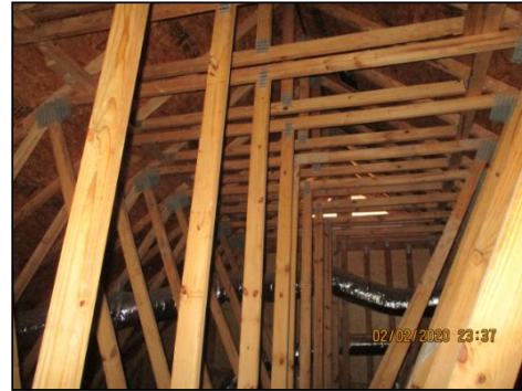
Engineered Trusses noted in good condition.
