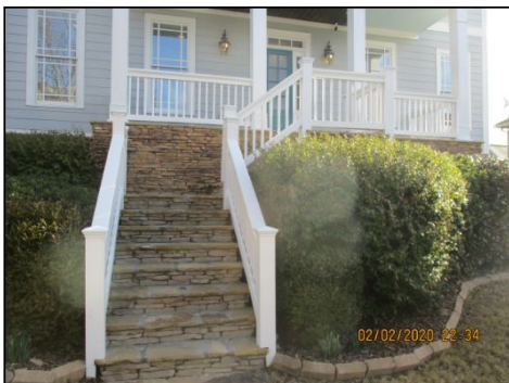
Stairs and handrails are in good condition.
