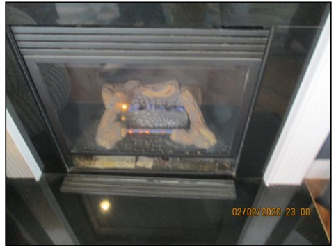
Gas fireplace with electric starter noted. Fireplace and hot box are in good condition.
