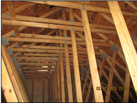
Engineered Trusses noted in good condition.
