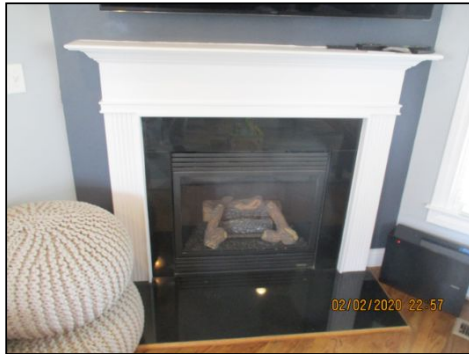
Gas fireplace with electric starter noted. Fireplace and hot box are in good condition.
