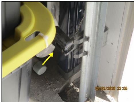
Eye beam system present and operating.
