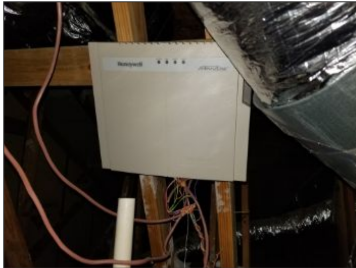
Dual zone thermostat control for HVAC system
