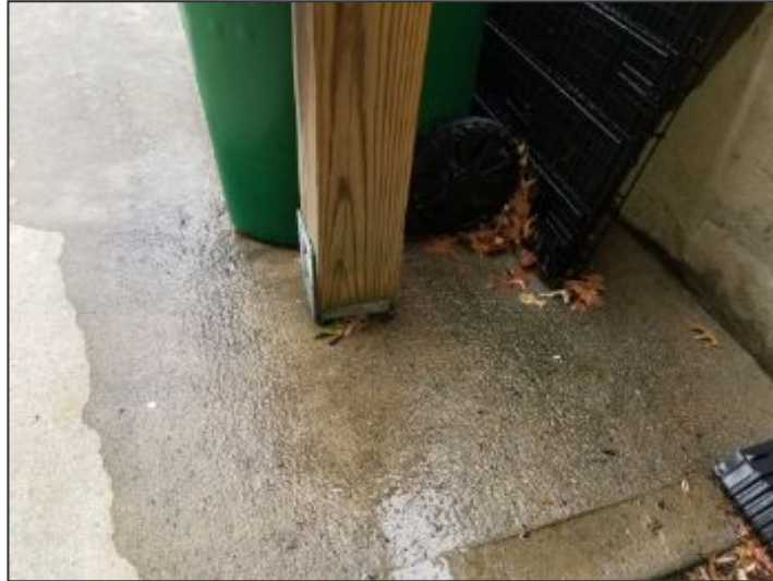
Good footing brackets at deck posts
