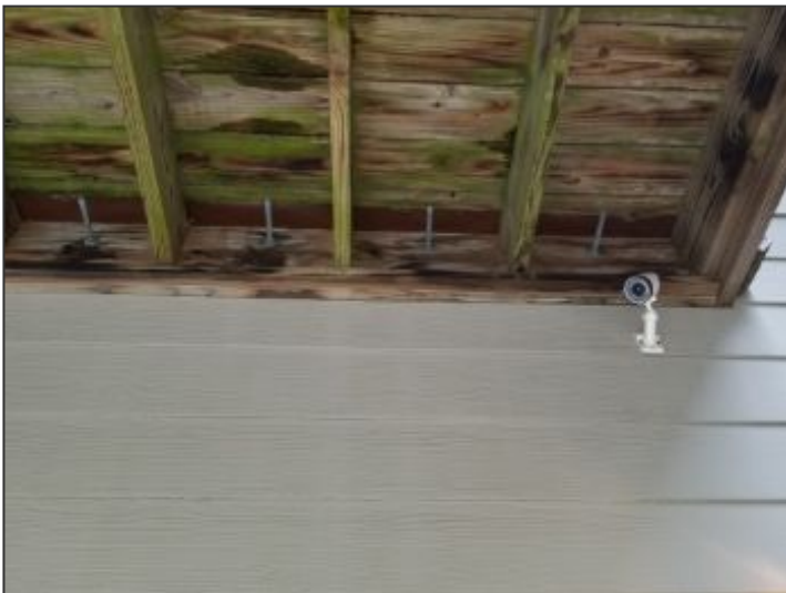
Good flashing, deck attachment and joist support at rear deck
