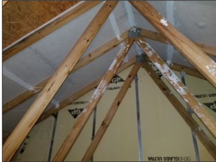
Good fire walls in attic
