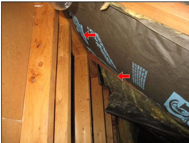
5.0 Item 2(Picture) Lower attic
