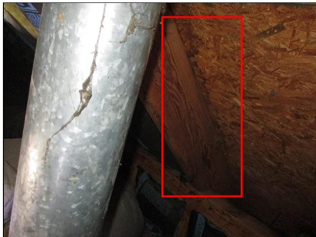
4.4 Item 1(Picture) lower attic
