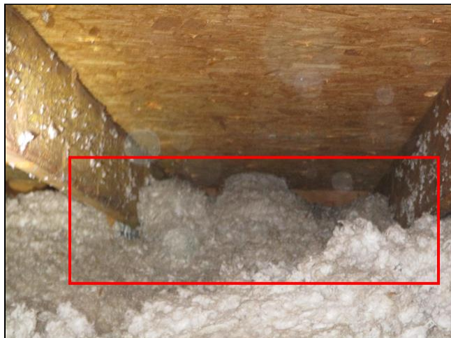
5.0 Item 4(Picture) upper attic
