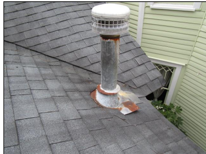
Prime and paint the flue assembly
