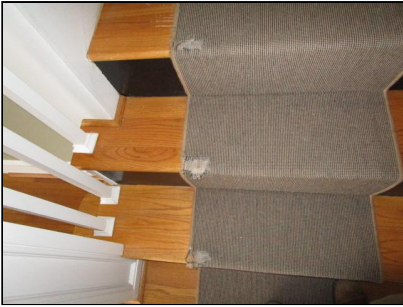
Carpet damaged, replace runner up the stairs.
