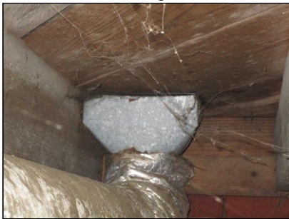
Add insulation to all register boots.
