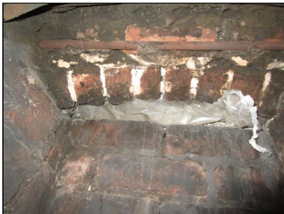
Some fireplaces blocked off.
