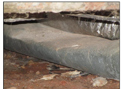
Repair damaged return duct, add insulation
