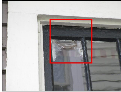
Replace cracked and damaged window panes.
