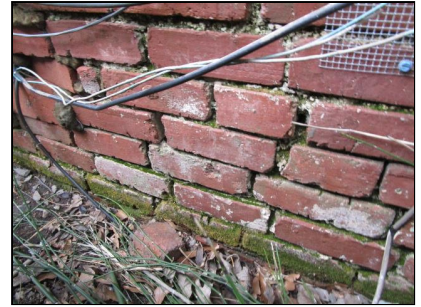
Scrape loose mortar on the exterior and repoint between bricks.
