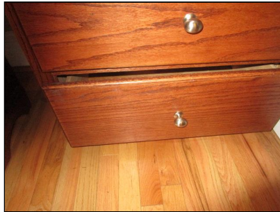
Repair drawers in the master bathroom
