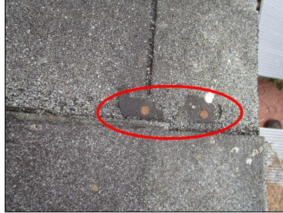
Seal exposed nail heads.
