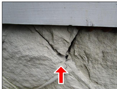
Repoint between stones where missing
