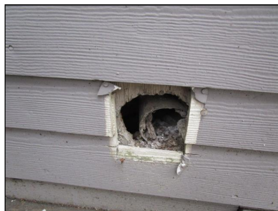
Secure dryer vent to new hood.
