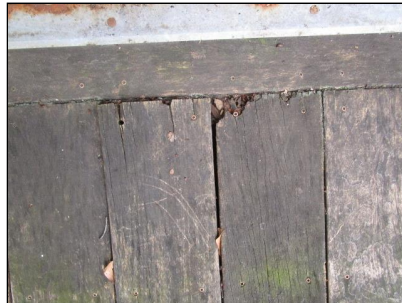
Replace damaged decking.
