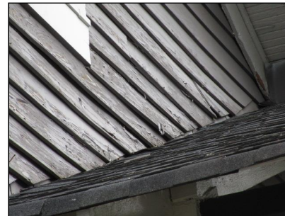
Paint weathered and peeling on the siding
