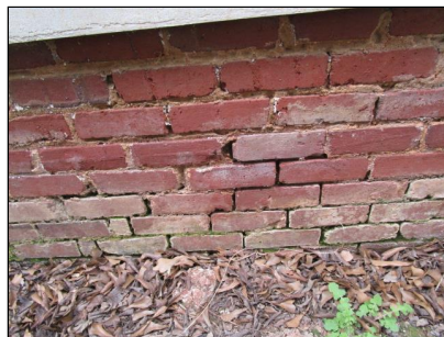
Scrape loose mortar on the exterior and repoint between bricks.
