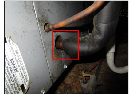
Add insulation and seal to the coil housing.
