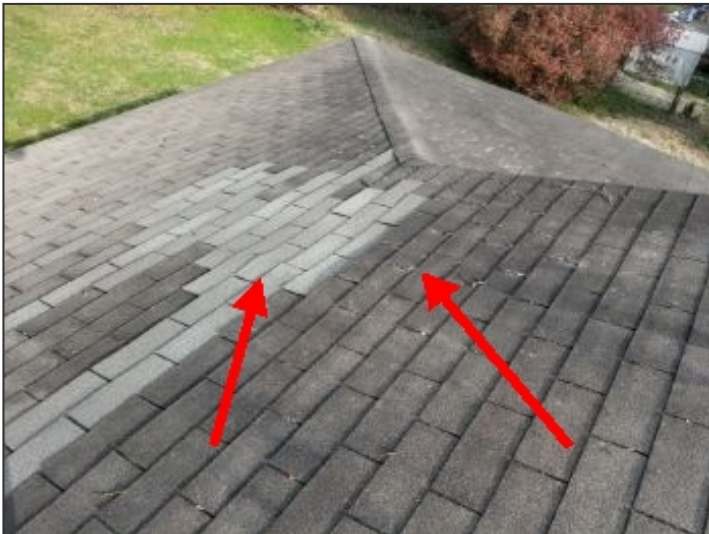
Shingle replacement at rear right roof and caulking repairs noted above
