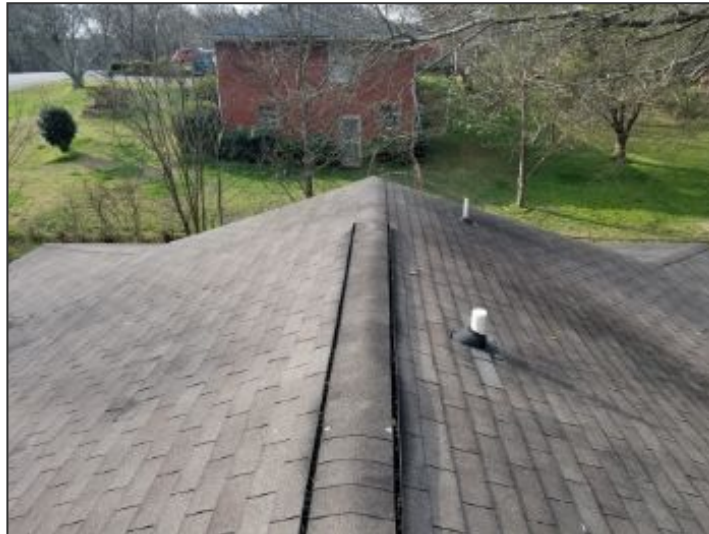
Walked roof during inspection
