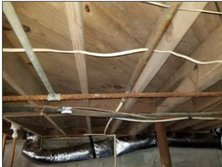
Recommend floor insulation in crawl space
