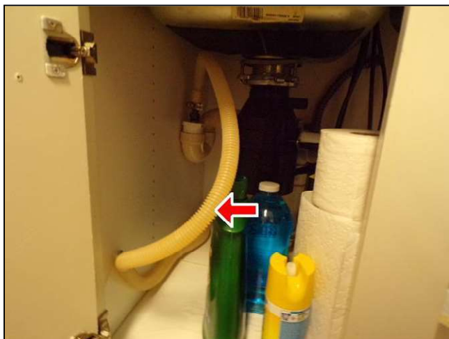
6.0 Under kitchen sink
