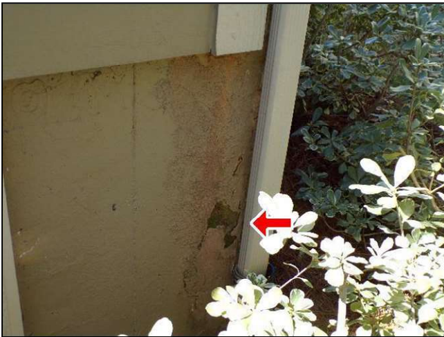
2.0 Rear of home foundation wall
