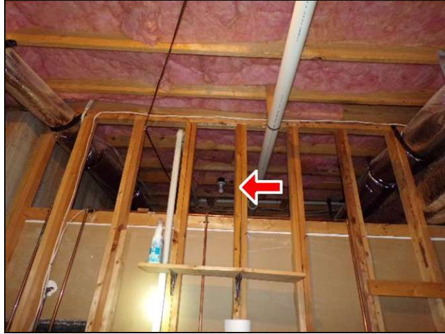
8.3 Upper area rear basement room
