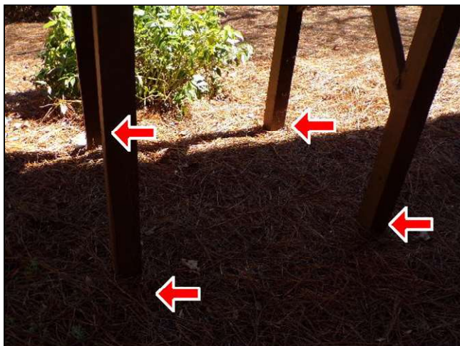
1.1 rear deck stair posts
