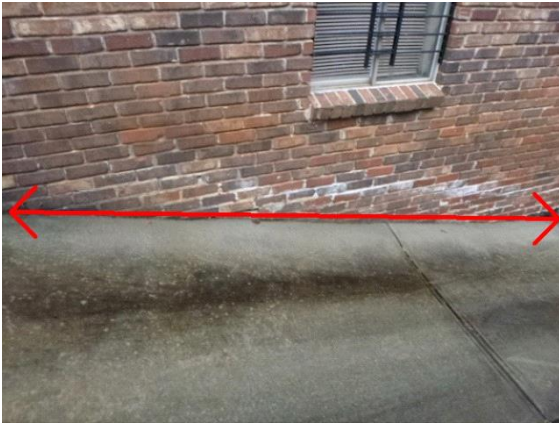
Foundation: seal gaps
