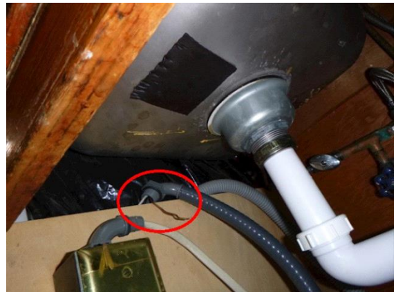
Kitchen: exposed splice
