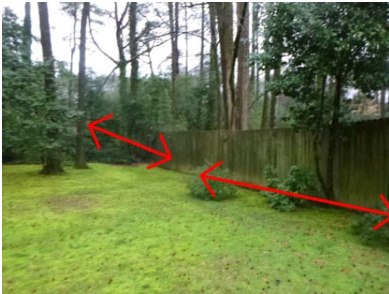
Fences / Gates: leaning, rotting
