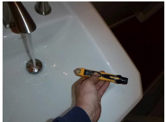
Hall Bathroom : water temp at 99F
