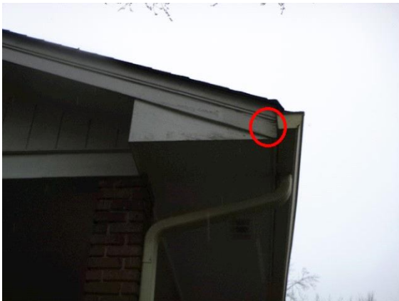
Exterior Surface: Wood rot
