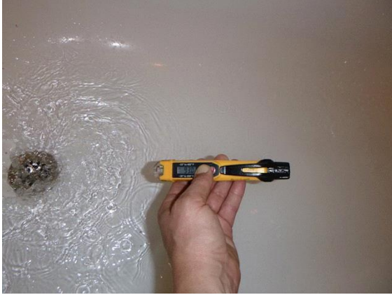
Hall Bathroom : shower water temp at 93F
