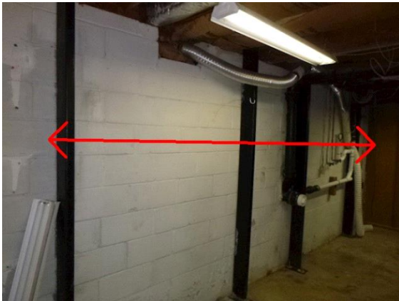
Interior Foundation: steel supports added
