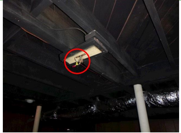
Electrical: exposed wiring
