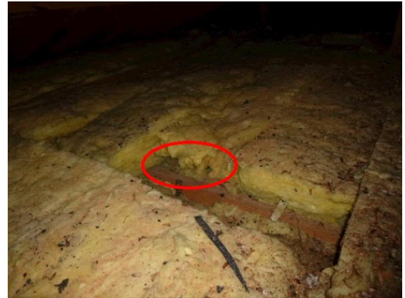
Attic Insulation: tunnels
