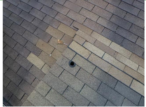
Roofing: vent flush with roof
