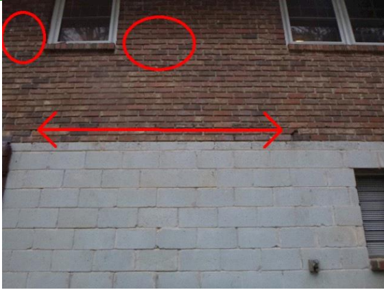
Exterior Surface: seal holes
