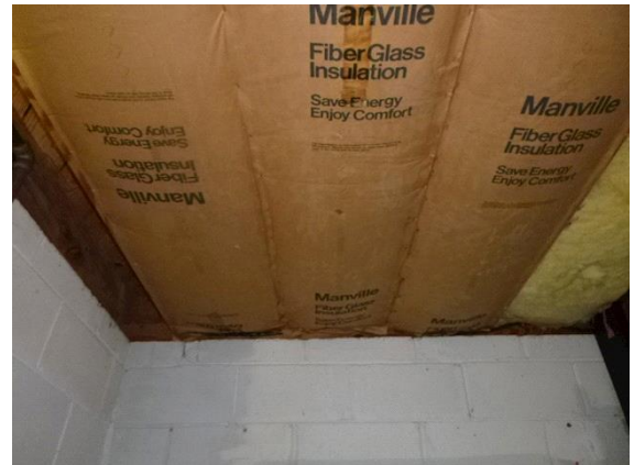
Under Floor Framing & Support: insulation facing exposed
