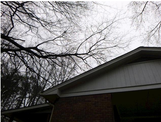
Roofing: Trim trees
