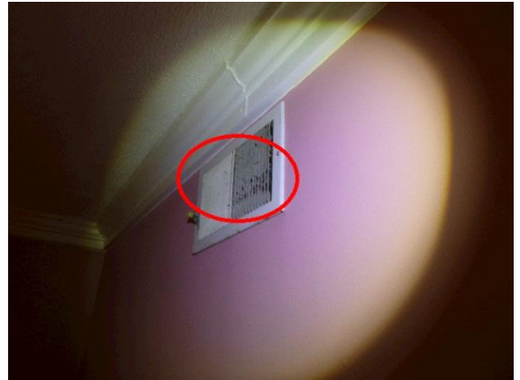
Under Floor Framing & Support: Suspected fungal growth
