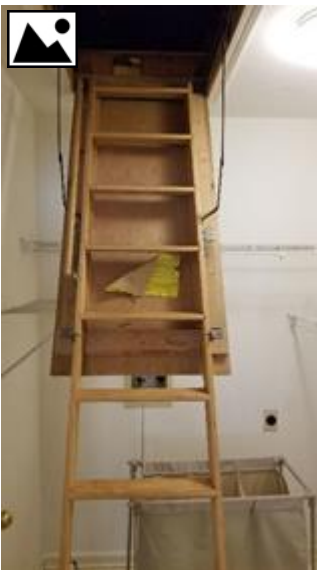
View from Attic Entry
