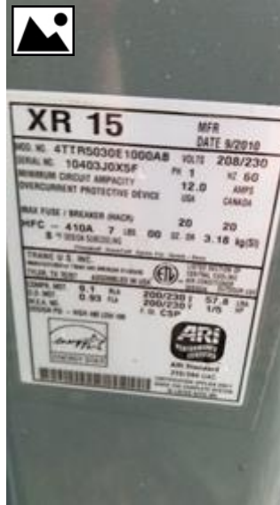
HVAC - Cooling System 2 Data Tag
